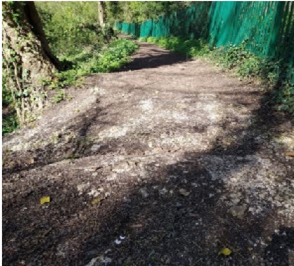
Bridleway adjacent Nicholson Road industrial estate
